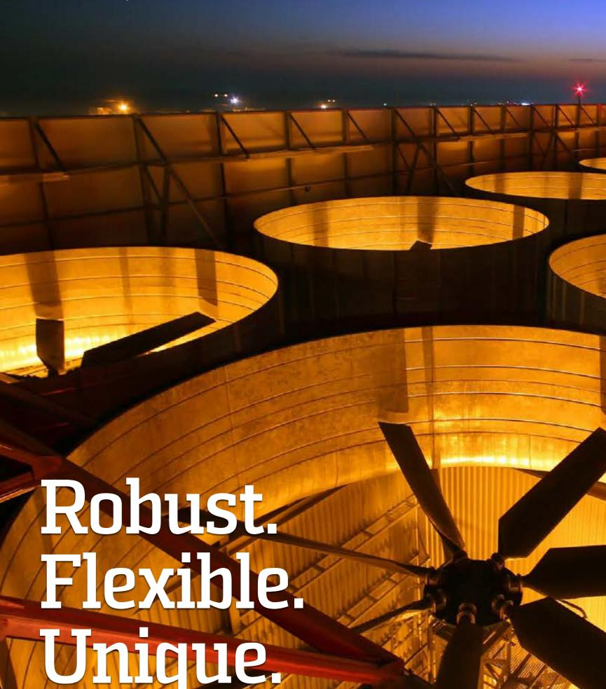
All parts can be protected against corrosion by either electroplated coating or paint, which protects the steel parts against aggressive media and environmental impacts.
